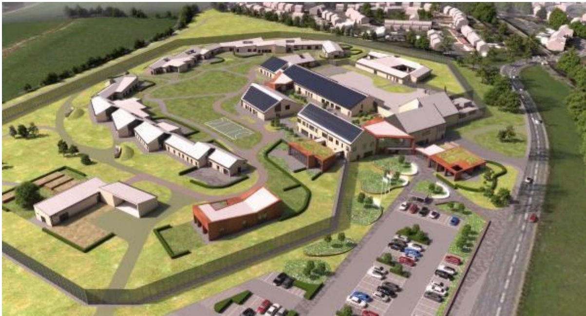
Aerial View of Women's National Facility
